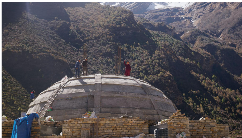
Geshe-la atop the World Peace Stupa, under construction, April 2025
